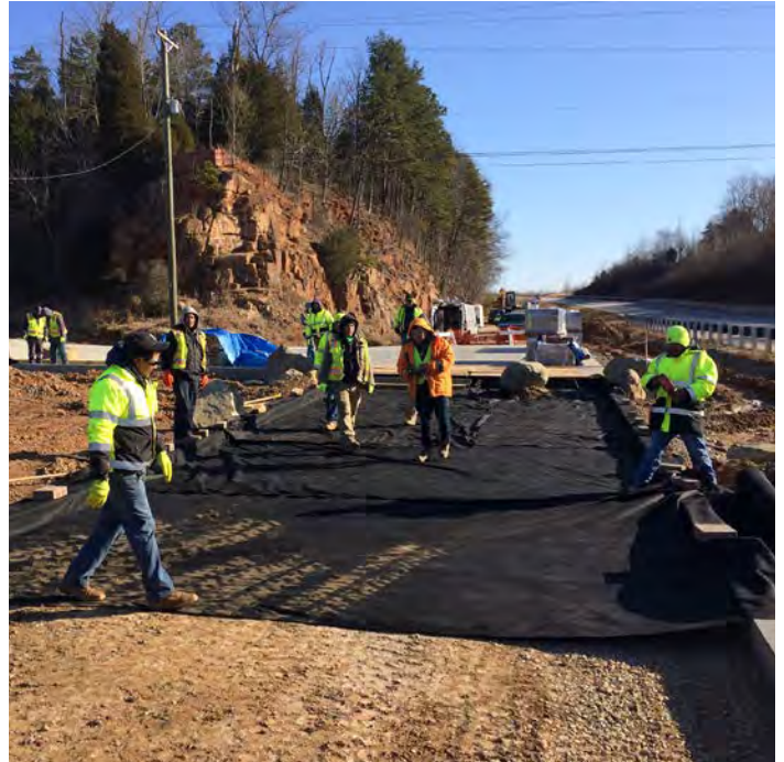
Yadkin River Park-Davidson County Trailhead during plaza construction
