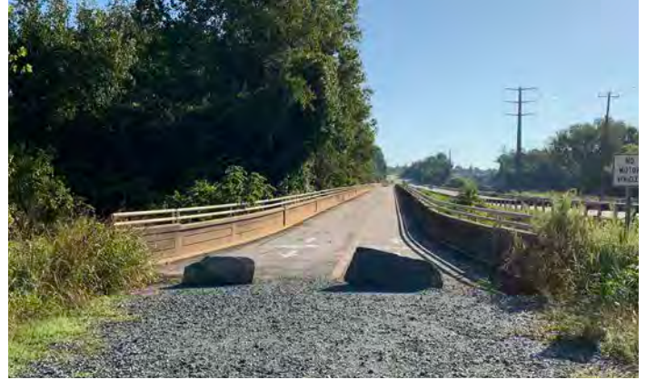
Site of future Yadkin River Park Rowan trailhead plaza
