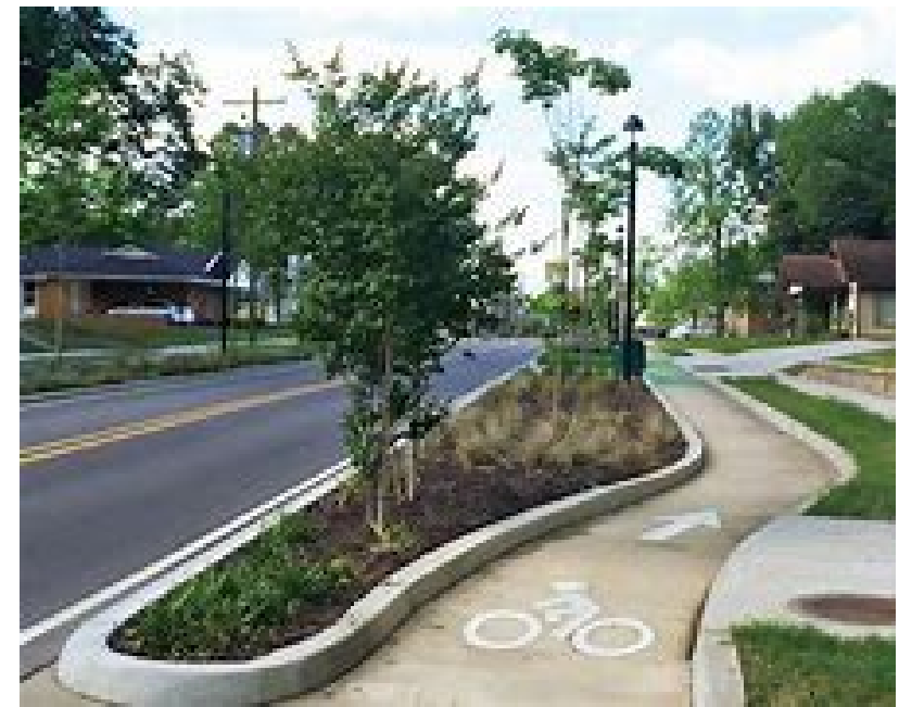
More elaborate bike lane with traffic calming bumpout
