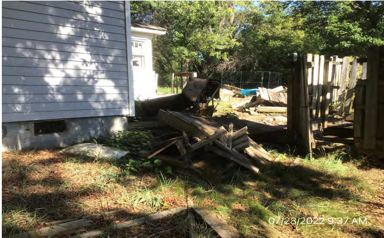
Exhibit A: 204 S. Iredell Ave Front Porch and yard condition before clean up
