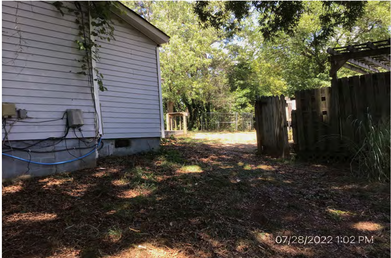
Exhibit B: 204 S. Iredell Ave After Clean-up
