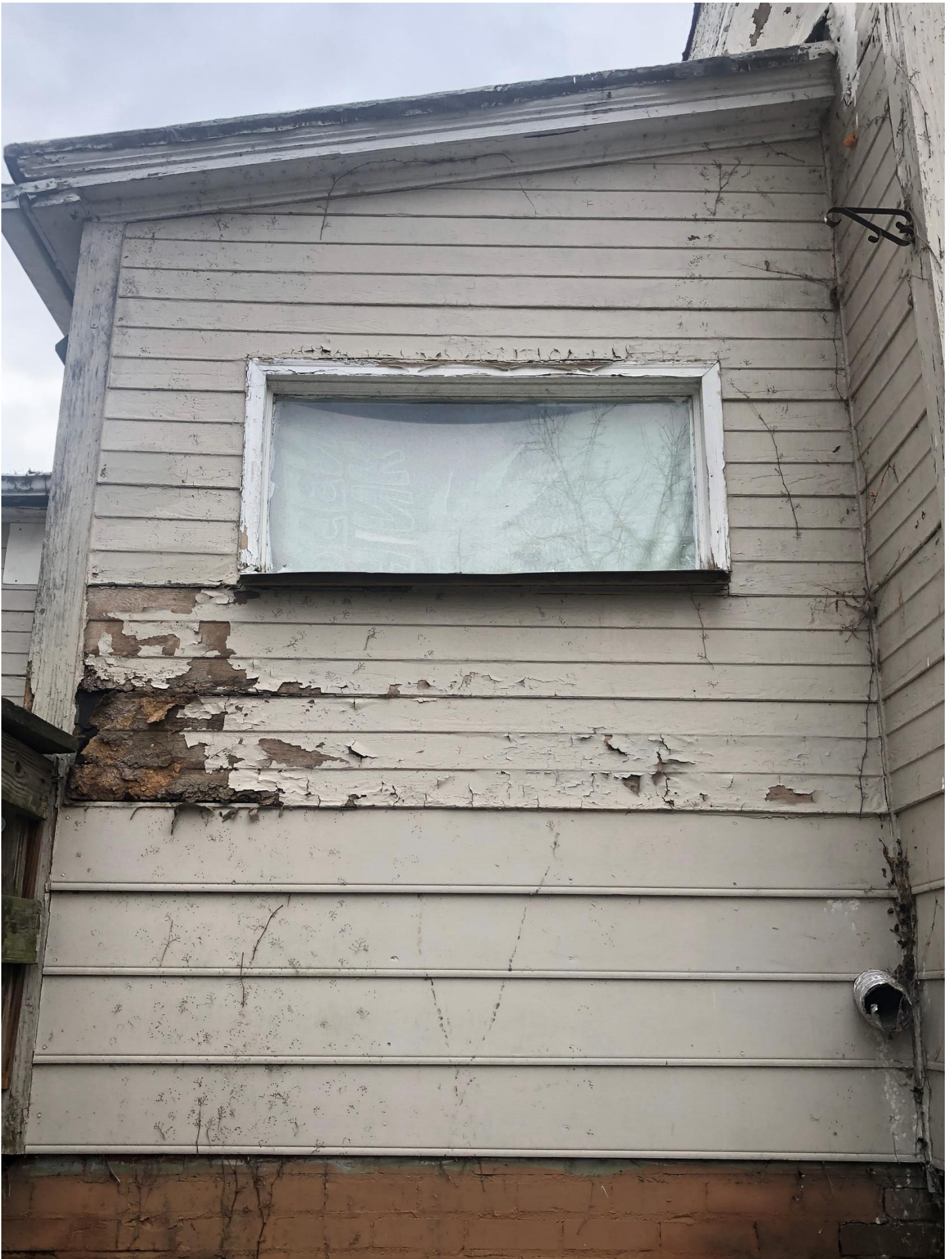
Exhibit A: Staff Photographs (Site Visit 1/19/23)
