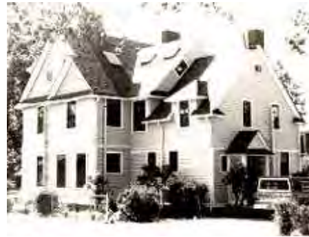
Non-obtrusive skylights on rear of residence.
