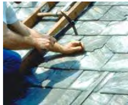
Repairing slate roof using traditional methods.
