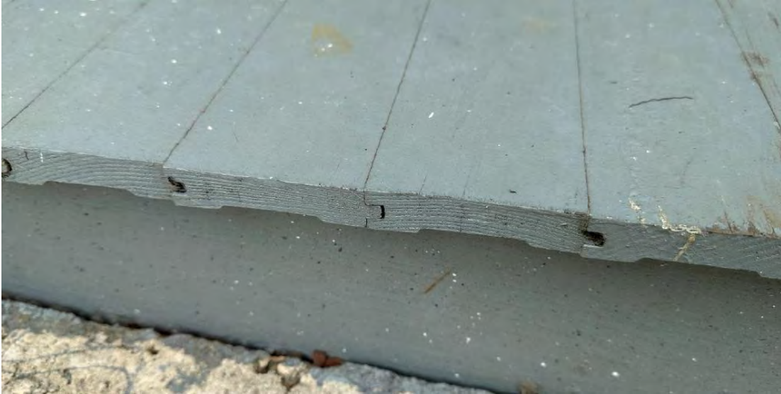
(Above) Existing wood T&G flooring.
