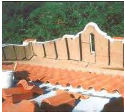
Replacement of damaged clay tile roof.
