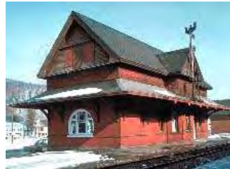
Gable and pent roof in excellent condition.
