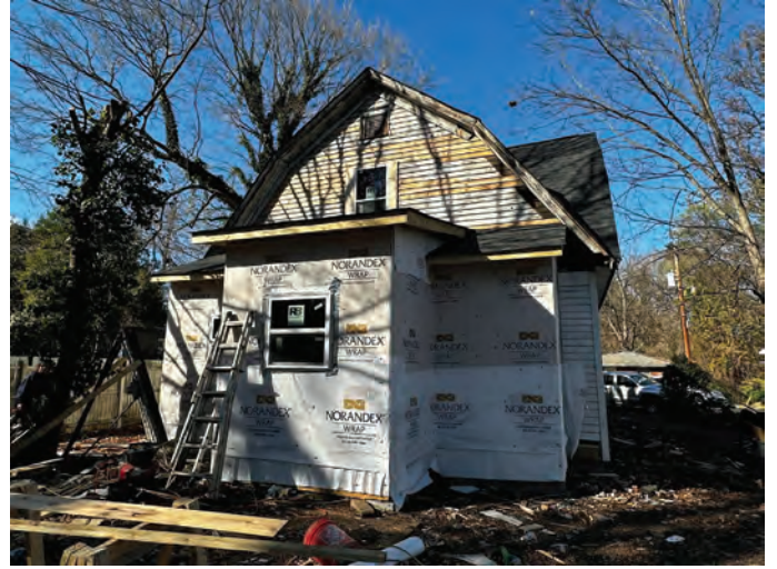
Exhibit B – Staff Photographs (Site Visit 11/28/2023)
