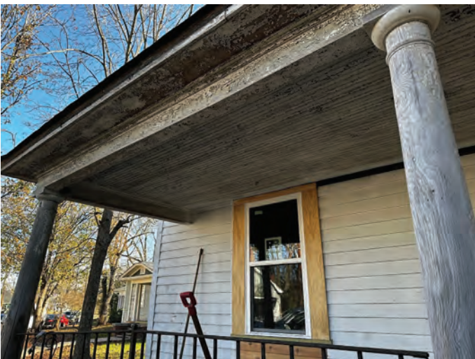
Exhibit B – Staff Photographs (Site Visit 11/28/2023)
