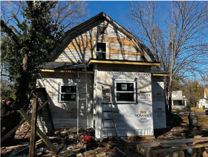
Exhibit B – Staff Photographs (Site Visit 11/28/2023)
