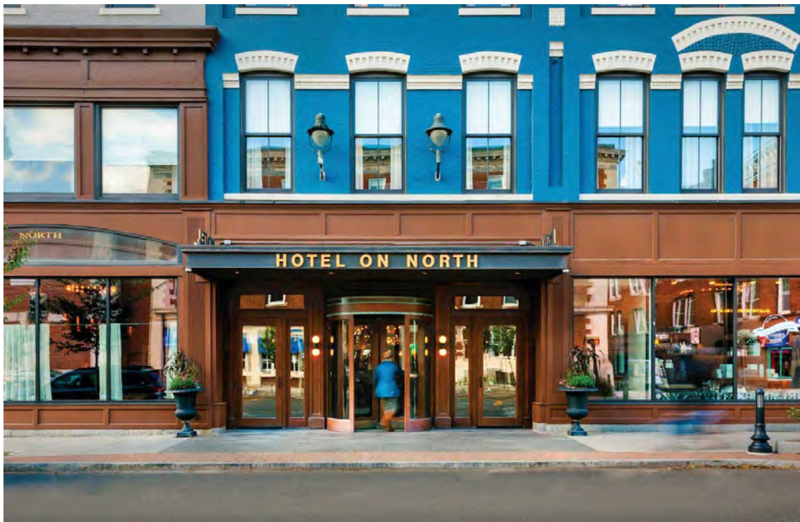
(Below) Marvin Clad Wood Double Hung Windows substantially replicate the appearance of original.
