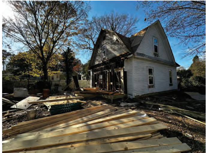
Exhibit A – Staff Photographs (Preliminary Site Investigation 11/6/2023)
