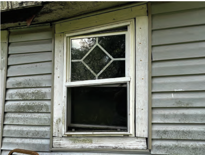
Exhibit A – Staff Photographs (Site Visit September 2023)
