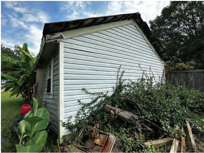
Exhibit A – Staff Photographs (Site Visit September 2023)
