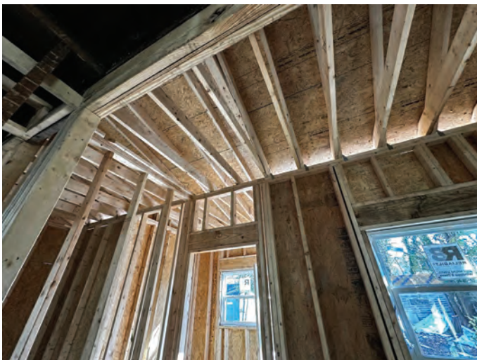
Exhibit B – Staff Photographs (Site Visit 11/28/2023)
