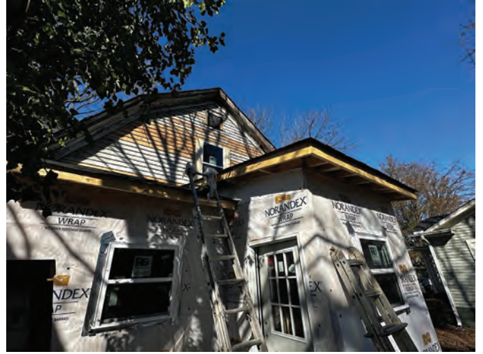
Exhibit B – Staff Photographs (Site Visit 11/28/2023)
