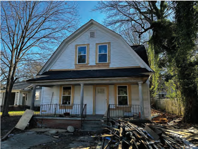
Exhibit B – Staff Photographs (Site Visit 11/28/2023)
