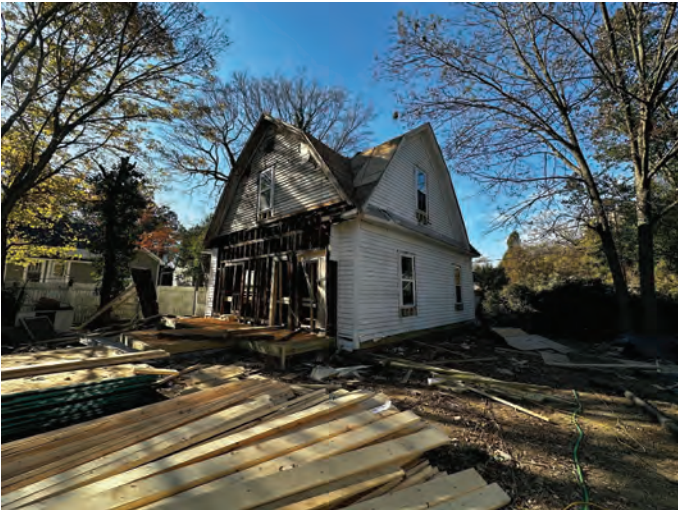
Exhibit A – Staff Photographs (Preliminary Site Investigation 11/6/2023)
