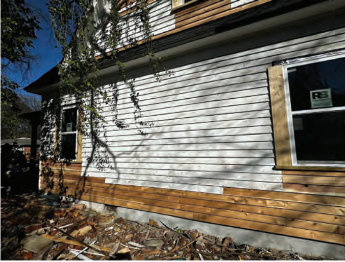
Exhibit B – Staff Photographs (Site Visit 11/28/2023)
