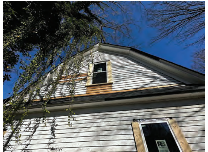
Exhibit B – Staff Photographs (Site Visit 11/28/2023)
