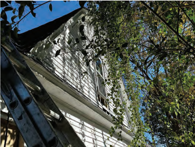
Exhibit A – Staff Photographs (Preliminary Site Investigation 11/6/2023)
