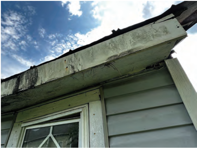
Exhibit A – Staff Photographs (Site Visit September 2023)
