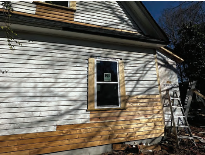
Exhibit B – Staff Photographs (Site Visit 11/28/2023)
