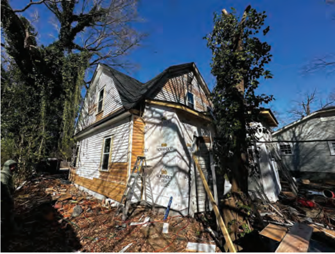
Exhibit B – Staff Photographs (Site Visit 11/28/2023)
