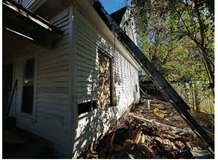
Exhibit A – Staff Photographs (Preliminary Site Investigation 11/6/2023)
