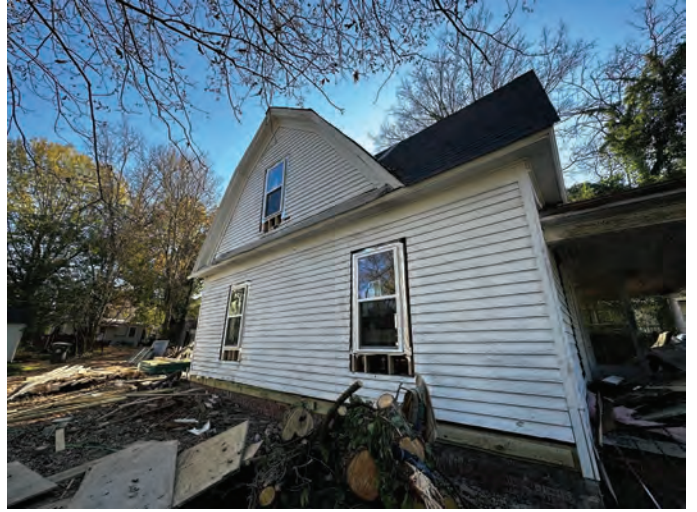
Exhibit A – Staff Photographs (Preliminary Site Investigation 11/6/2023)
