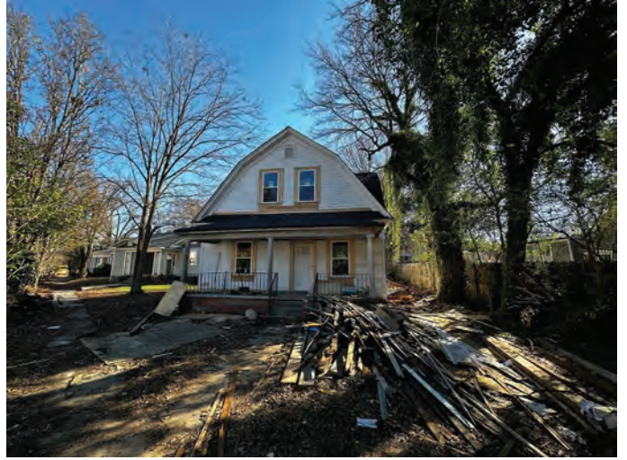
Exhibit B – Staff Photographs (Site Visit 11/28/2023)
