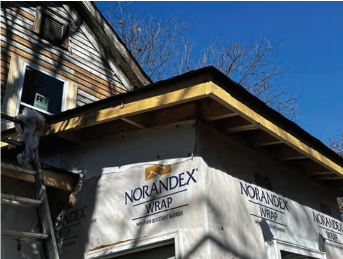
Exhibit B – Staff Photographs (Site Visit 11/28/2023)
