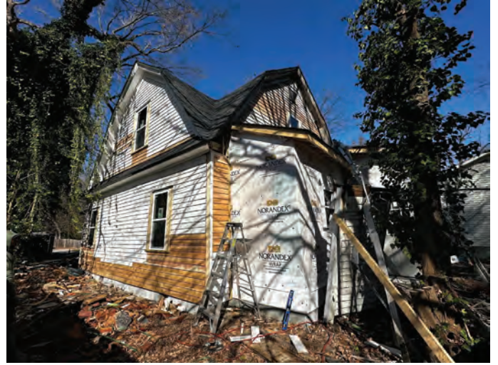
Exhibit B – Staff Photographs (Site Visit 11/28/2023)
