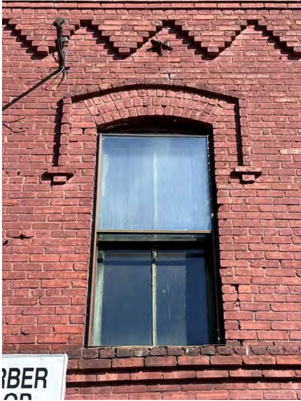
Example of older wood window on adjacent building(s)
