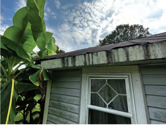
Exhibit A – Staff Photographs (Site Visit September 2023)
