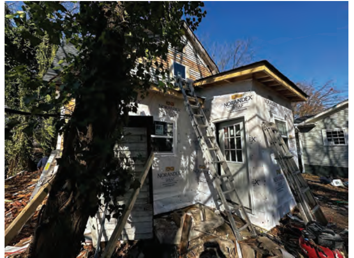
Exhibit B – Staff Photographs (Site Visit 11/28/2023)
