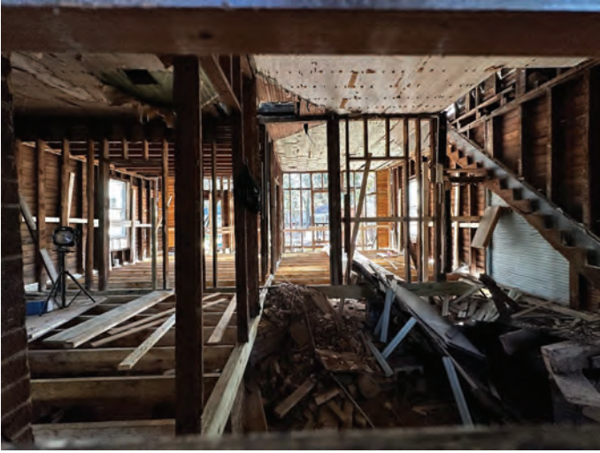
Exhibit A – Staff Photographs (Preliminary Site Investigation 11/6/2023)
