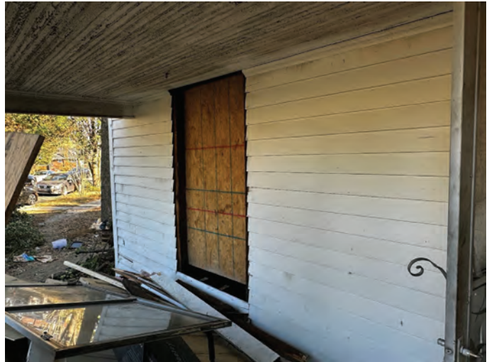
Exhibit A – Staff Photographs (Preliminary Site Investigation 11/6/2023)
