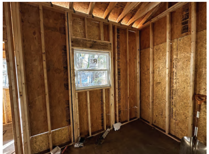
Exhibit B – Staff Photographs (Site Visit 11/28/2023)
