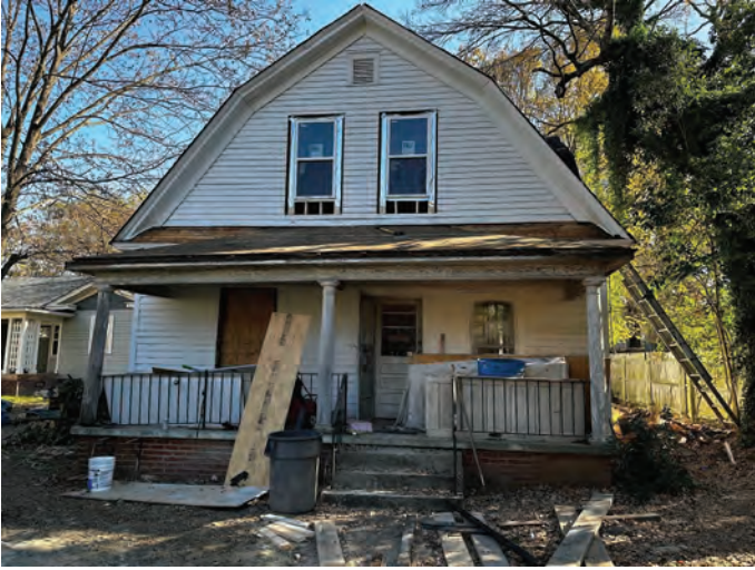
Exhibit A – Staff Photographs (Preliminary Site Investigation 11/6/2023)
