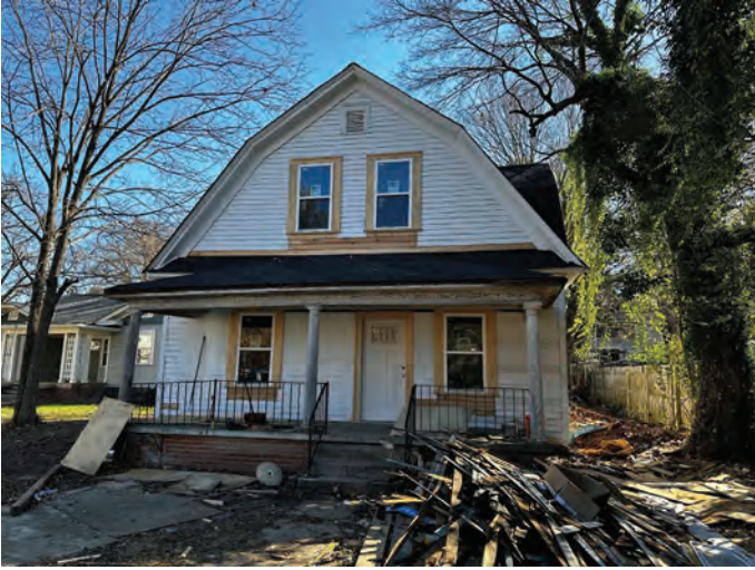
Exhibit B – Staff Photographs (Site Visit 11/28/2023)
