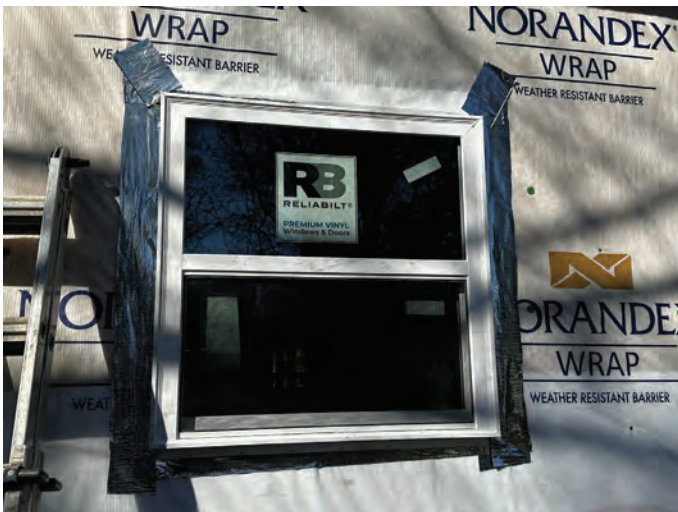
Exhibit B – Staff Photographs (Site Visit 11/28/2023)
