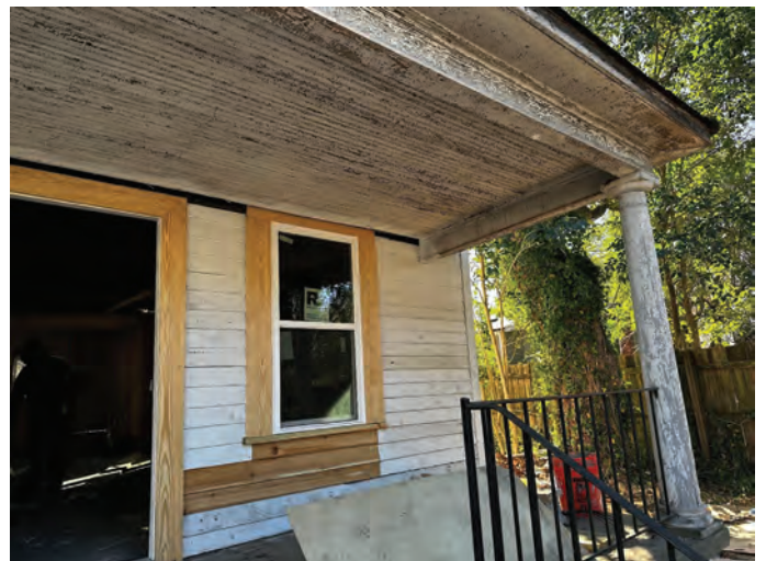
Exhibit B – Staff Photographs (Site Visit 11/28/2023)
