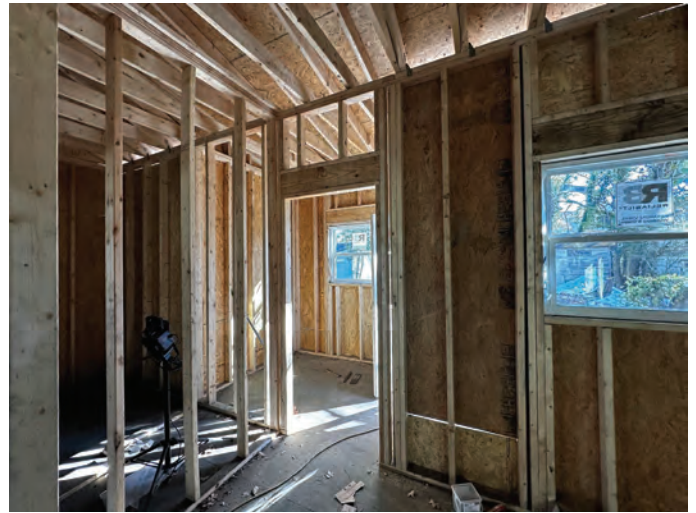
Exhibit B – Staff Photographs (Site Visit 11/28/2023)
