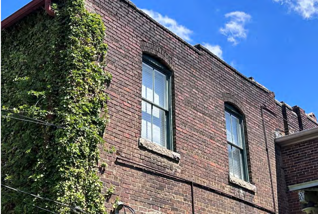
(Above) Original 2-over-2 wood windows remain on the rear of the subject building.
