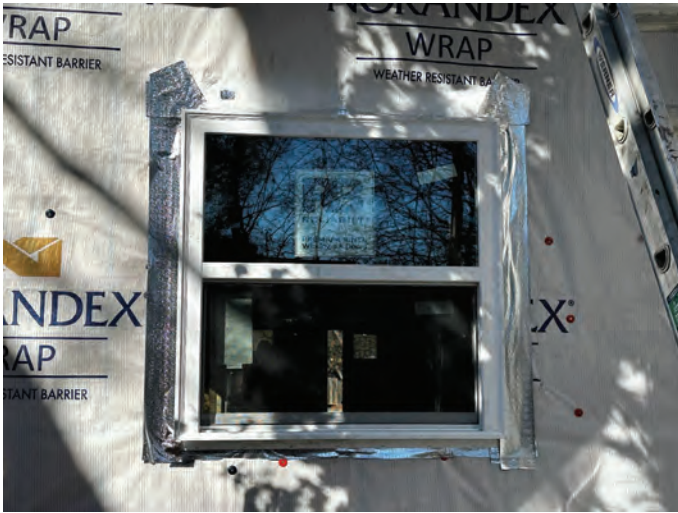
Exhibit B – Staff Photographs (Site Visit 11/28/2023)
