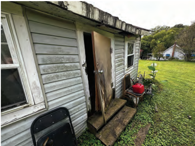
Exhibit A – Staff Photographs (Site Visit September 2023)
