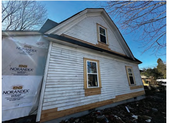
Exhibit B – Staff Photographs (Site Visit 11/28/2023)
