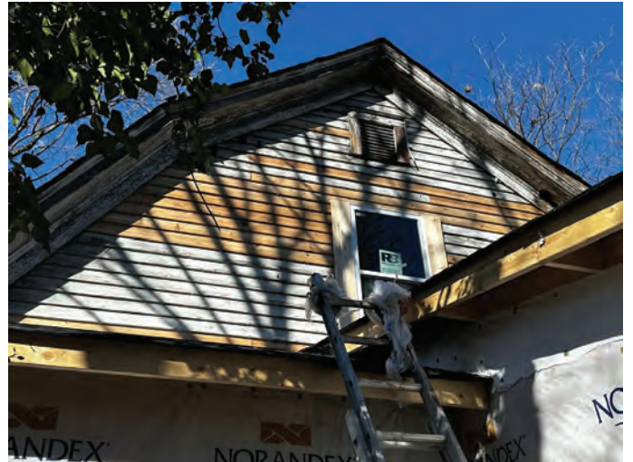
Exhibit B – Staff Photographs (Site Visit 11/28/2023)
