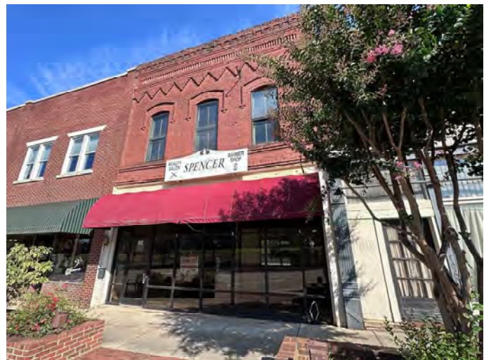
Example of older wood window on adjacent building(s)
