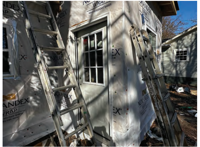
Exhibit B – Staff Photographs (Site Visit 11/28/2023)
