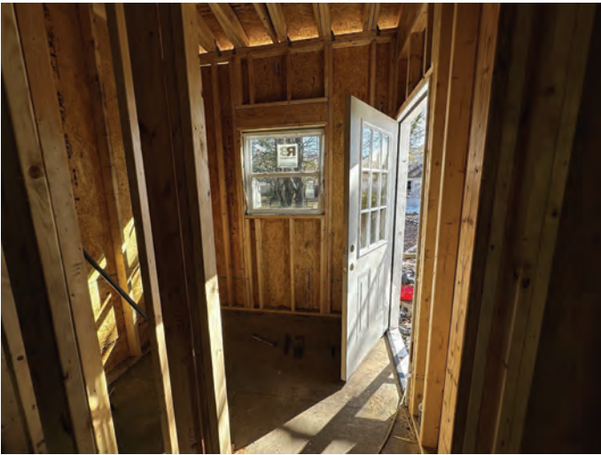
Exhibit B – Staff Photographs (Site Visit 11/28/2023)
