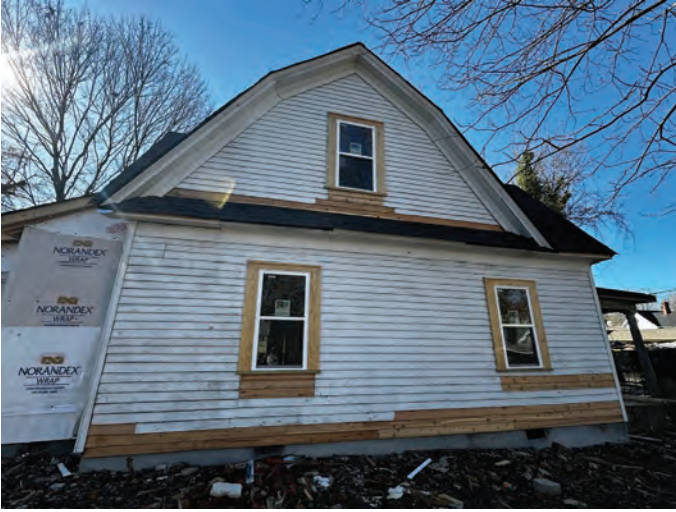
Exhibit B – Staff Photographs (Site Visit 11/28/2023)
