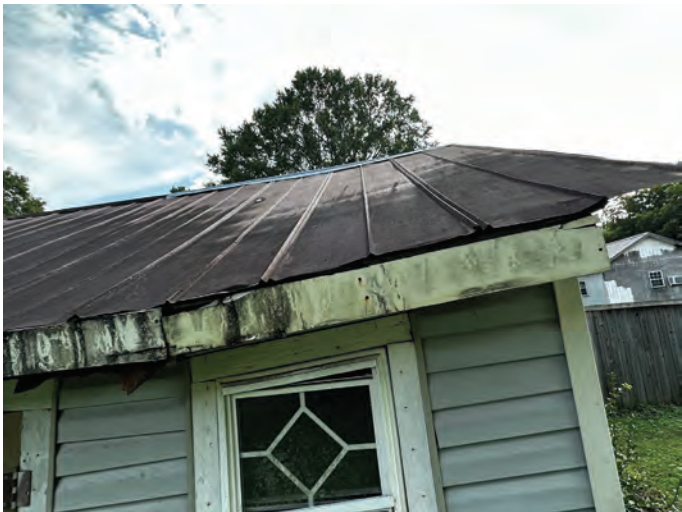
Exhibit A – Staff Photographs (Site Visit September 2023)
