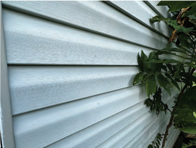
Exhibit A – Staff Photographs (Site Visit September 2023)
