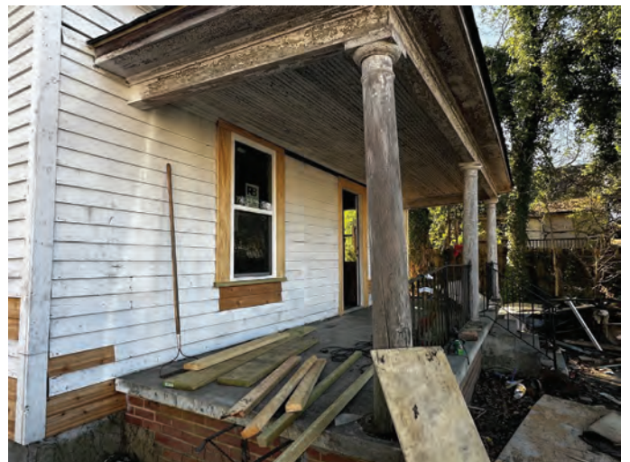
Exhibit B – Staff Photographs (Site Visit 11/28/2023)
