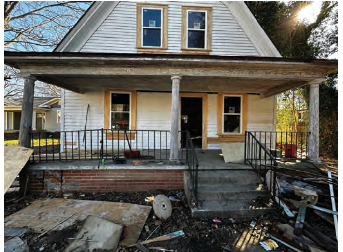
Exhibit B – Staff Photographs (Site Visit 11/28/2023)
