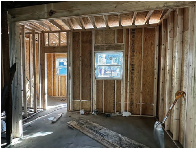
Exhibit B – Staff Photographs (Site Visit 11/28/2023)
