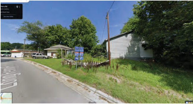
View Looking west down Long Ferry
