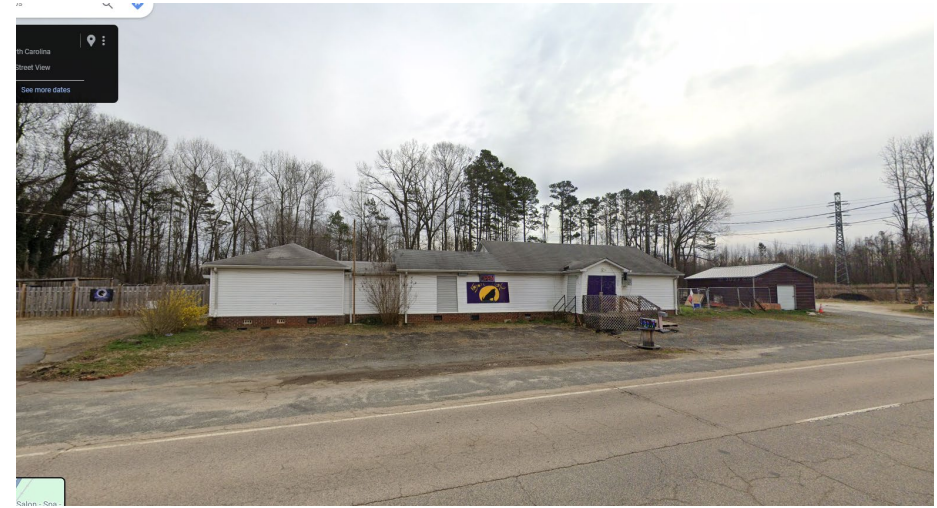
Existing Commercial Structure
