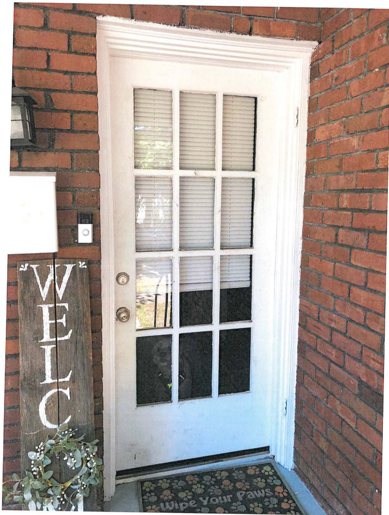
Exhibit C: Property & Door Photographs
