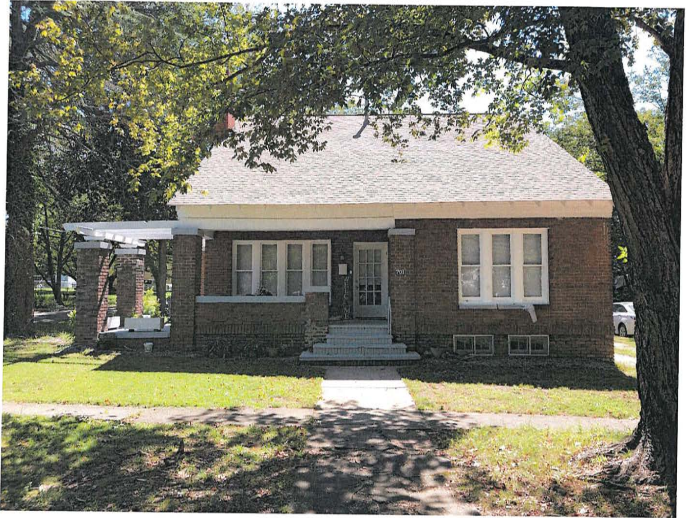
Exhibit C: Property & Door Photographs
