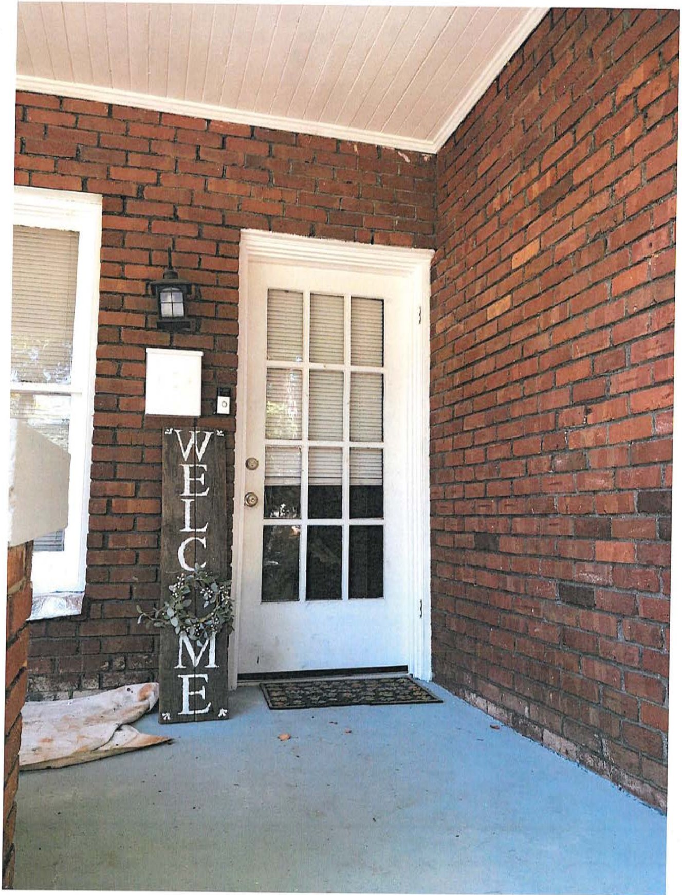
Exhibit C: Property & Door Photographs
