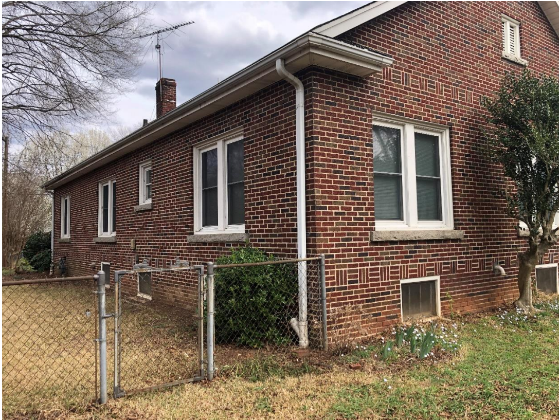
View of Right-Side Elevation (more photographs in Exhibit A):
