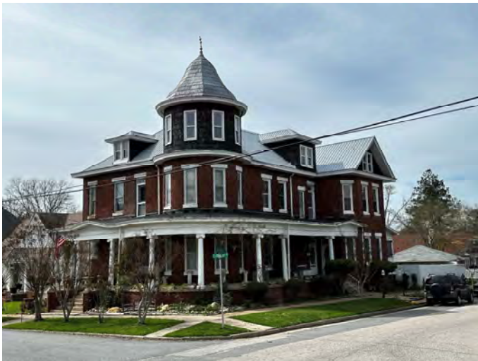
Figure 3 Roof Detail (New Standing Seam Metal Panels). Site Visit 3-25-2024 by Kyle Harris, HPC Liaison.
