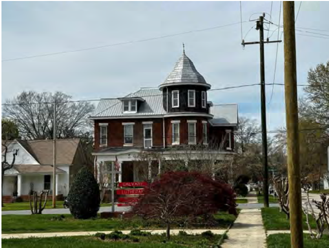
Figure 1 Roof Detail (New Standing Seam Metal Panels). Site Visit 3-25-2024 by Kyle Harris, HPC Liaison.
