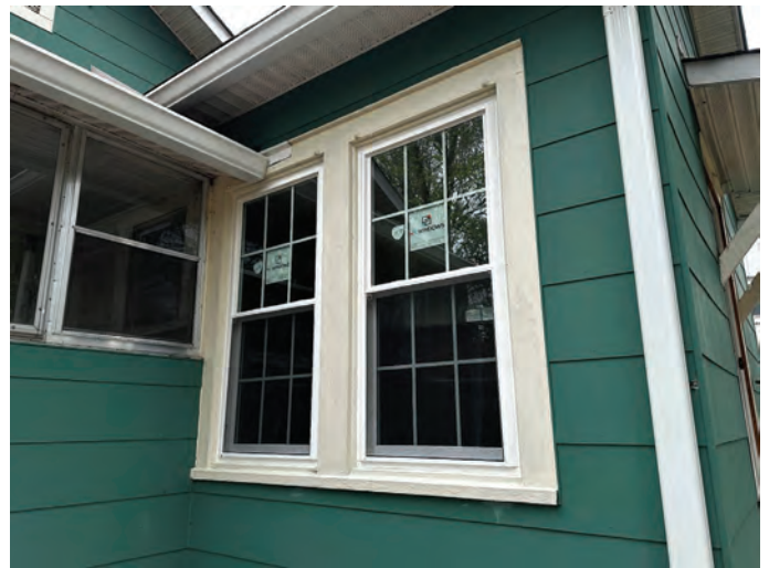
Figure 12 Window Detail (New Vinyl Replacement Windows). Site Visit 3-26-2024 by Kyle Harris, HPC Staff Liaison.
