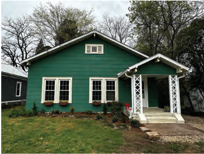
Figure 1 Window Detail (New Vinyl Replacement Windows). Site Visit 3-26-2024 by Kyle Harris, HPC Staff Liaison.
