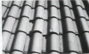
Repairs on this panicle roof were made with new tiles held in place with metal hangers. (Main Building, Ellis Island, New York)
