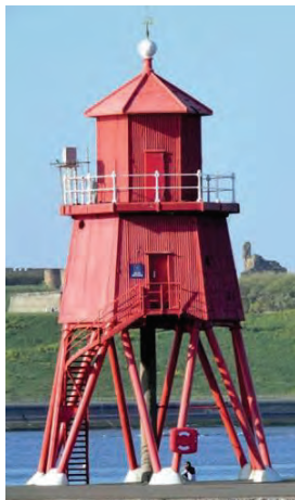
Herd Groyne Lighthouse (1881), South Shields, Tyne and Wear (Photo: Emma Joyce)
