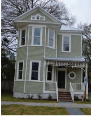
505 Ann Street, front (south) façade (3/16/2022)
