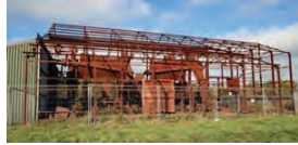
The significance of a building is not always apparent from its appearance. Stripped of its corrugated iron cladding, this early 20th-century structure forms part of a peat processing plant and is a rare survivor of an industry dating back to medieval times. The structure is Grade II* listed and a scheduled ancient monument.
