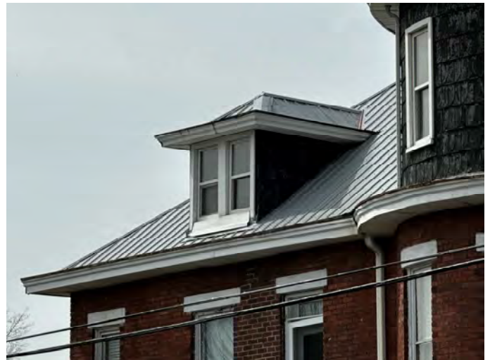
Figure 4 Roof Detail (New Standing Seam Metal Panels). Site Visit 3-25-2024 by Kyle Harris, HPC Liaison.
