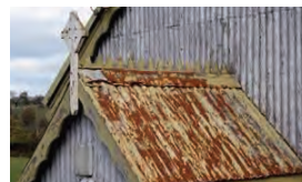
Regular painting is often all that is needed to ensure that iron cladding remains in good condition. Simple features such as this decorative ridge piece require particular attention to ensure the character of the building is preserved.
