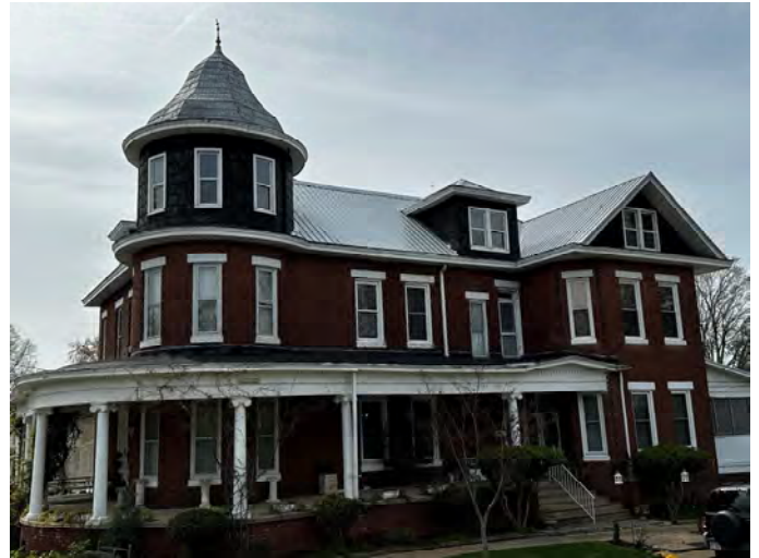
Figure 6 Roof Detail (New Standing Seam Metal Panels). Site Visit 3-25-2024 by Kyle Harris, HPC Liaison.
