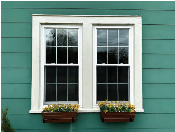
Figure 3 Window Detail (New Vinyl Replacement Windows). Site Visit 3-26-2024 by Kyle Harris, HPC Staff Liaison.
