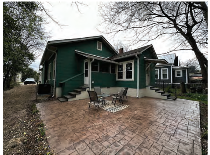
Figure 10 Window Detail (New Vinyl Replacement Windows). Site Visit 3-26-2024 by Kyle Harris, HPC Staff Liaison.
