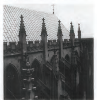
Good design and quality materials for the roof surface, fastenings, and flashing minimize roofing failures. This is essential on roofs such as on the National Cathedral where a thorough maintenance inspection and minor repairs cannot be done easily without special scaffolding. However, the success of the roof on any structure depends on frequent cleaning and repair of the gutter system. (Washington, D.C., photo courtesy of John Burns, A. I. A.)
