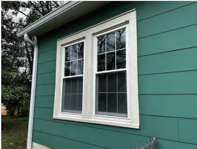
Figure 7 Window Detail (New Vinyl Replacement Windows). Site Visit 3-26-2024 by Kyle Harris, HPC Staff Liaison.
