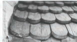
Replacement of particular historic details is important to the individual historic character of a roof, such as the treatment at the eaves of this rounded butt wood shingle roof. Also note that the surface of the roof was carefully sloped to drain water away from the side of the dormer. In the restoration, this function was augmented with the addition of carefully concealed modern metal flashing. (Mount Vernon, Virginia)
