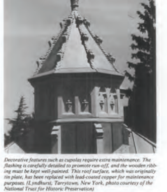
Decorative features such as cupolas require extra maintenance. The flashing is carefully detailed to promote run-off, and the wooden ribbing must be kept well-painted. This roof surface, which was originally tin plates, has been replaced with lead-coated copper for maintenance purposes. (Lynchburg, Tarrytown, New York, photo courtesy of the National Trust for Historic Preservation)
