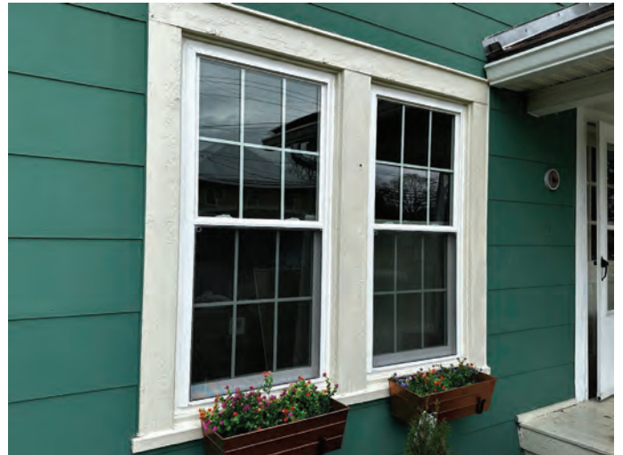
Figure 4 Window Detail (New Vinyl Replacement Windows). Site Visit 3-26-2024 by Kyle Harris, HPC Staff Liaison.
