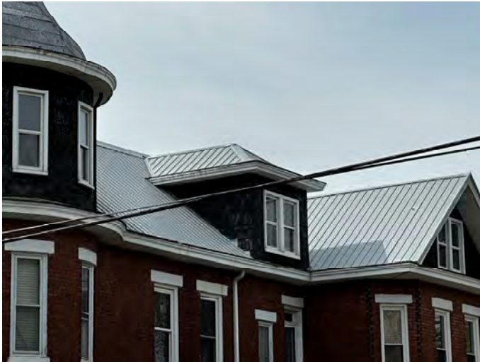
Figure 5 Roof Detail (New Standing Seam Metal Panels). Site Visit 3-25-2024 by Kyle Harris, HPC Liaison.
