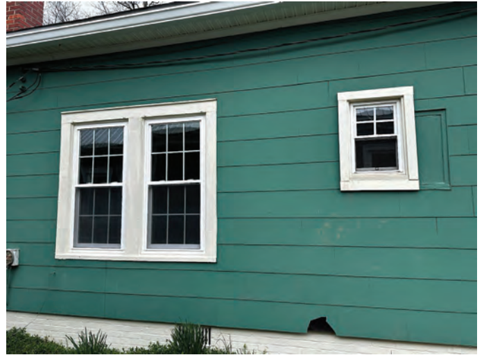
Figure 6 Window Detail (New Vinyl Replacement Windows). Site Visit 3-26-2024 by Kyle Harris, HPC Staff Liaison.
