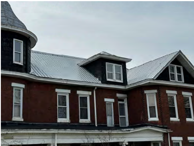
Figure 7 Roof Detail (New Standing Seam Metal Panels). Site Visit 3-25-2024 by Kyle Harris, HPC Liaison.
