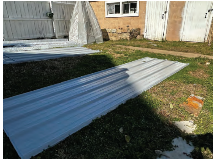
Figure 2 Site Visit 2-21-24 by Kyle Harris, HPC Liaison. Shown above: New standing seam metal panel, individual panel.
