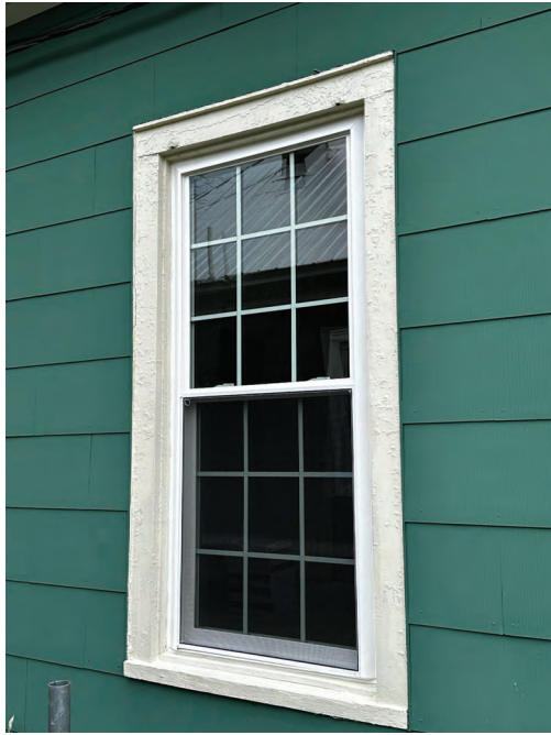
Figure 5 Window Detail (New Vinyl Replacement Windows). Site Visit 3-26-2024 by Kyle Harris, HPC Staff Liaison.
