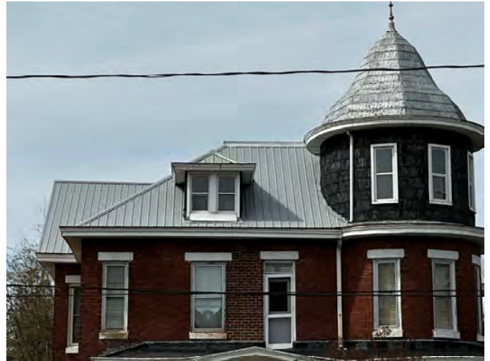
Figure 2 Roof Detail (New Standing Seam Metal Panels). Site Visit 3-25-2024 by Kyle Harris, HPC Liaison.
