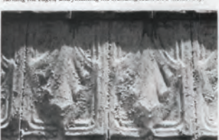
Tin shingles, commonly embossed to imitate wood or tile, or with a decorative design, were popular as an inexpensive, textured roofing material. These shingles 4 1/2 inch by 12 1/2 inch on the exposed surface were designed with interlocking edges, but they have been repaired by surface nailing, which may cause future leakage. (Ballard House, Yorktown, Virginia, photo by Gordie Whittington, National Park Service)
