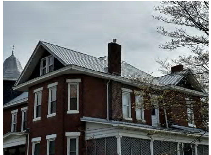
Figure 8 Roof Detail (New Standing Seam Metal Panels). Site Visit 3-25-2024 by Kyle Harris, HPC Liaison.
