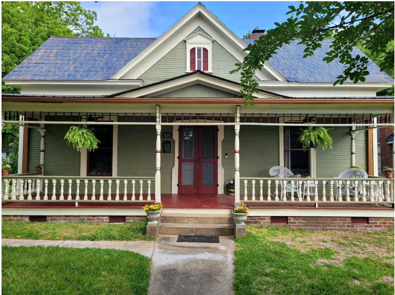
Existing Roof is Embossed Tin Shingle
